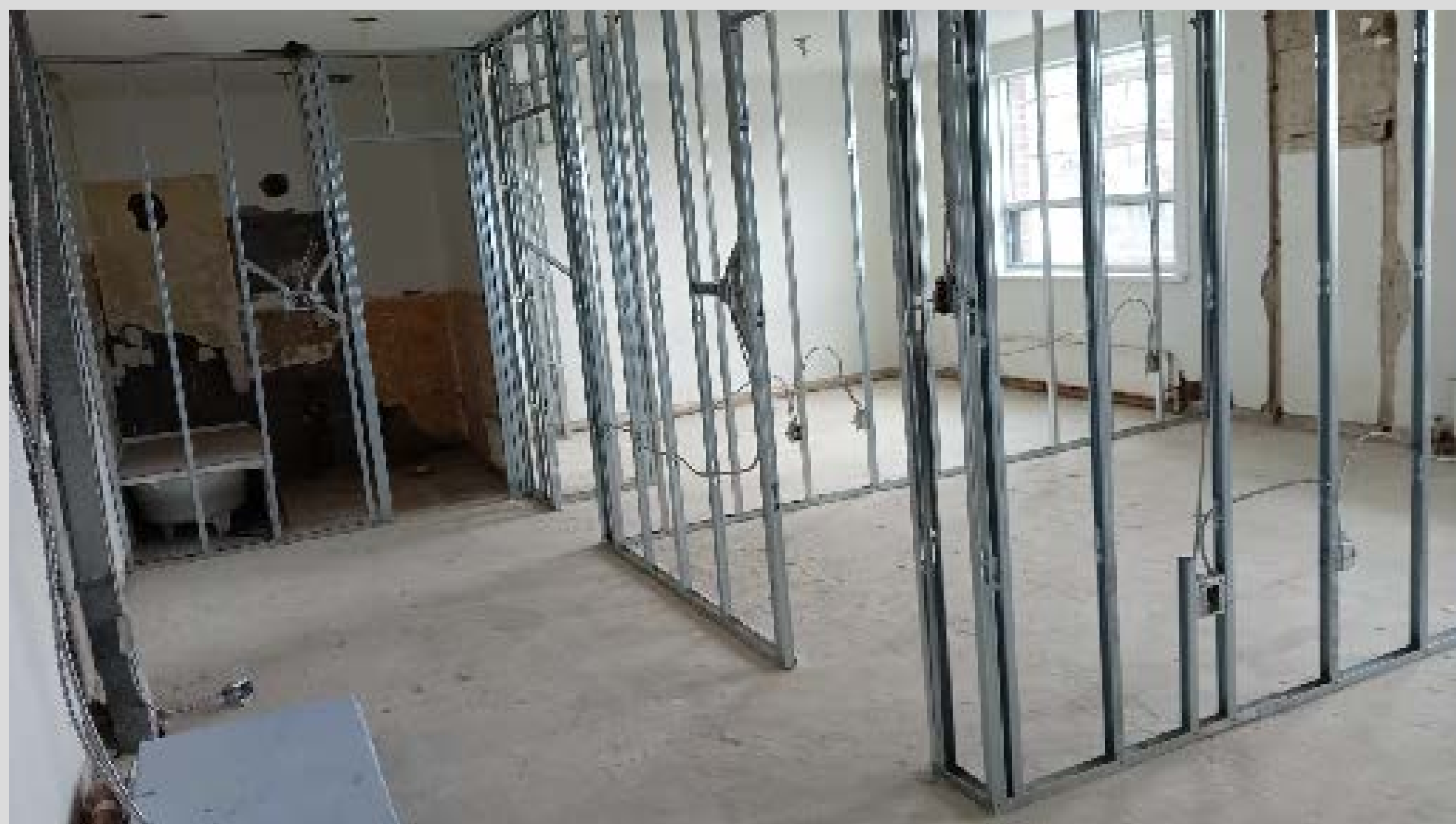
Rental unit demolition and metal framing
