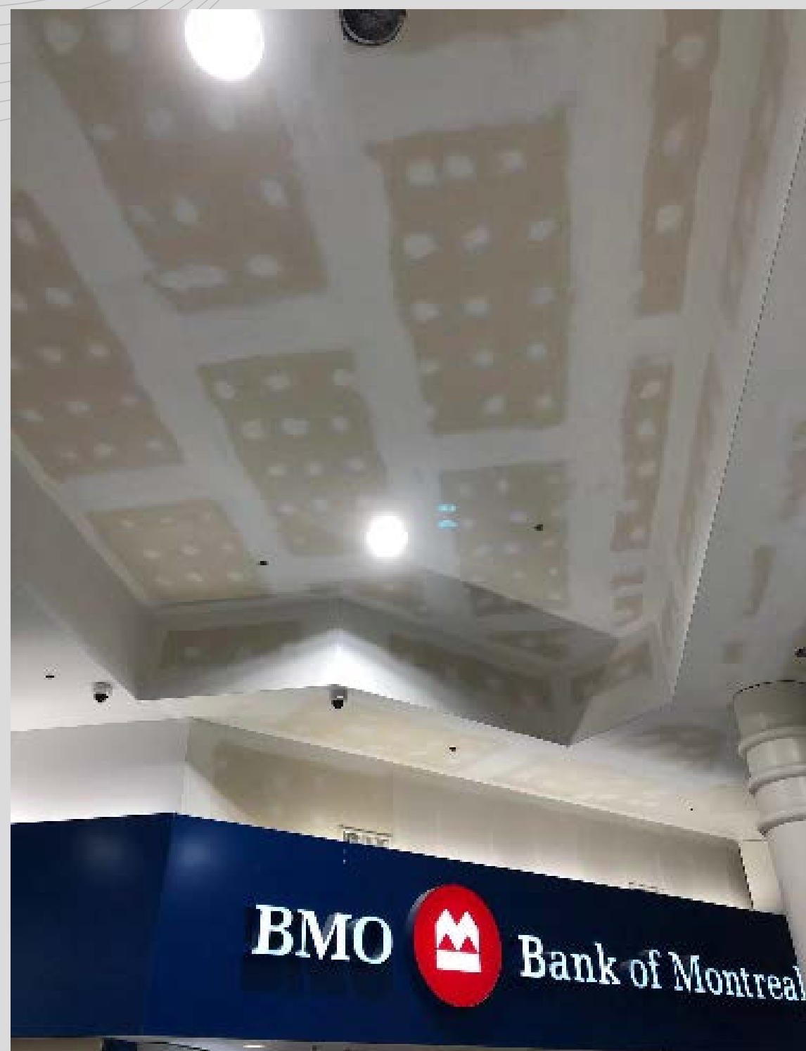
Drywall installation, tape and mudding
